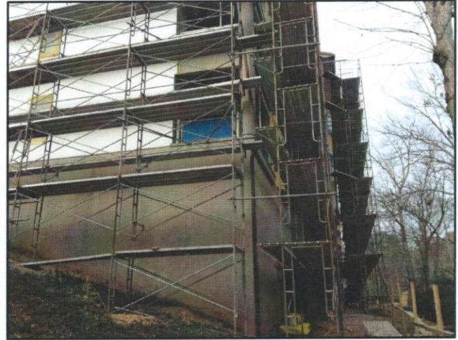
EIFS veneer system foam board insulation is being installed on the east end.
