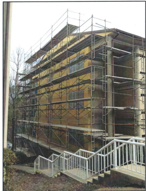
Water resistive coating has been applied over the entire building work area.
