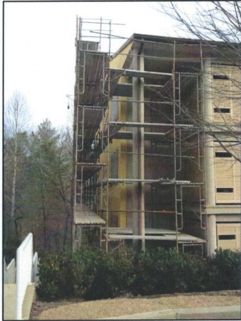
Repair work at front tall columns and corner walls is in progress.
