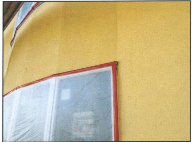
Selected views of water resistive coating with new windows installed at rear bow window walls.
