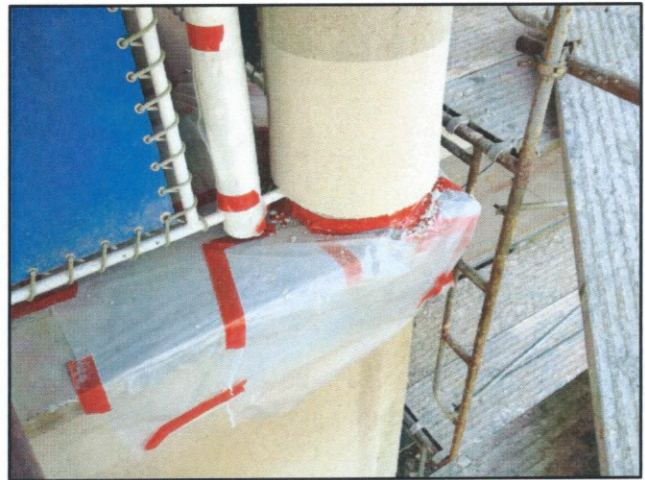
Private balcony corner column wood repairs are complete. Concrete floor and curbs are being installed. Stucco is being reapplied at the base of the columns.
