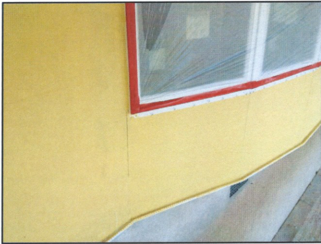
Selected views of water resistive coating with new windows installed at rear bow window walls.
