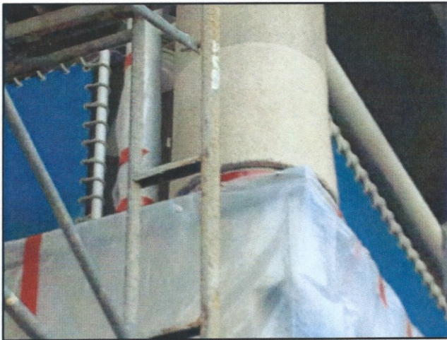
Private balcony corner column wood repairs are complete. Concrete floor and curbs are being installed. Stucco is being reapplied at the base of the columns.
