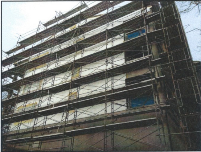
EIFS veneer system foam board insulation is being installed on the east end.
