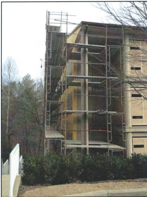
Water resistive coating has been applied over the entire building work area.
